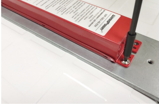
3. Attach battery driver to bracket.
